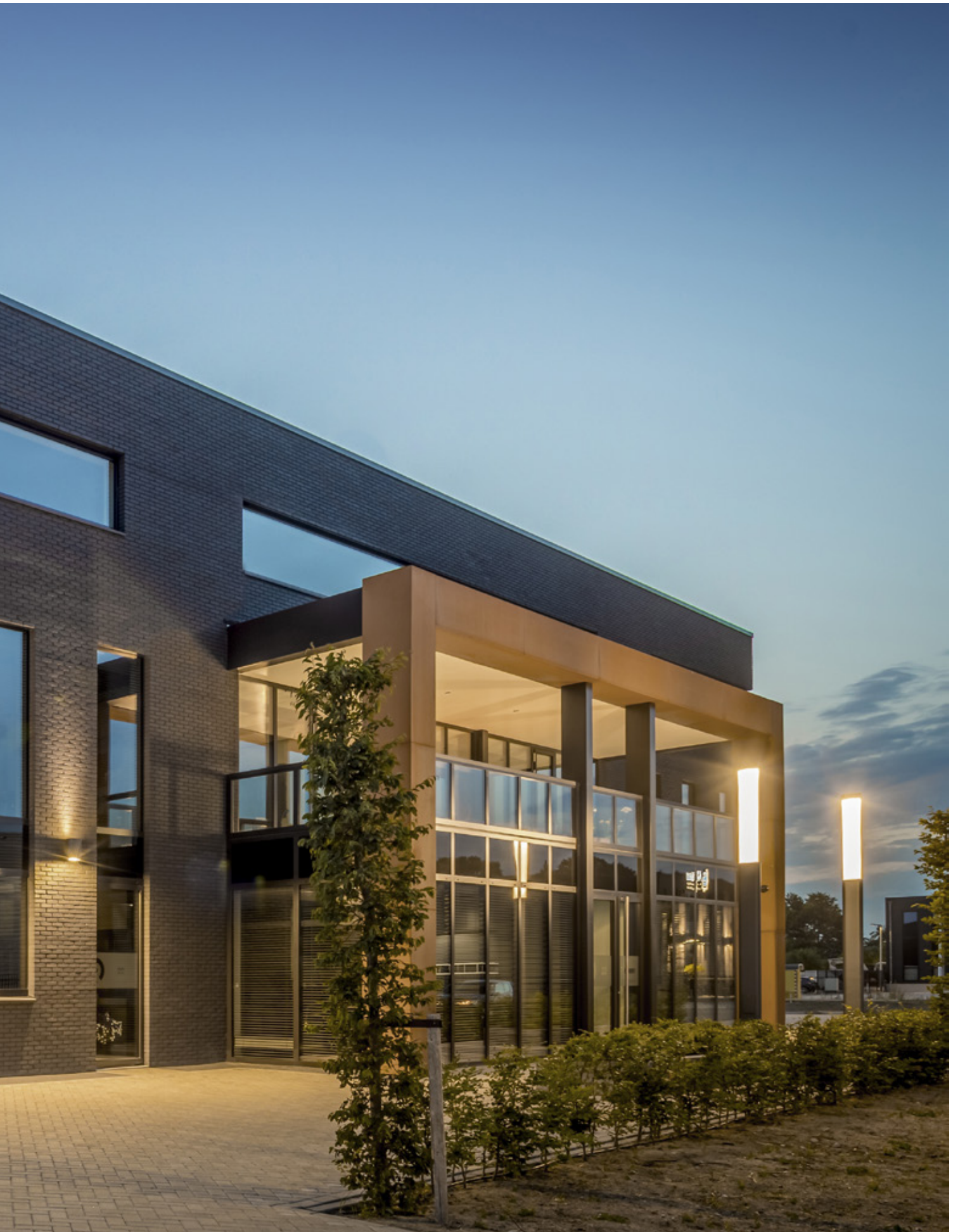
New building electrical wholesaler Robri | Wekerom | Netherlands
